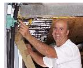
Nick puts the finishing touches on TWC's lawn irrigation system.
